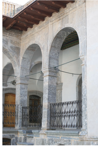
Fig. 14. Gypsum was extensively used on external surfaces of rich town-houses on the citadel of Erbil (photograph: author, 2016)
