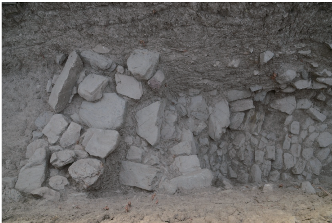
Fig. 7.5 Northern wall of the third stone structure (left) and the stair-like structure to the right in Operation D-2 (from the west)
