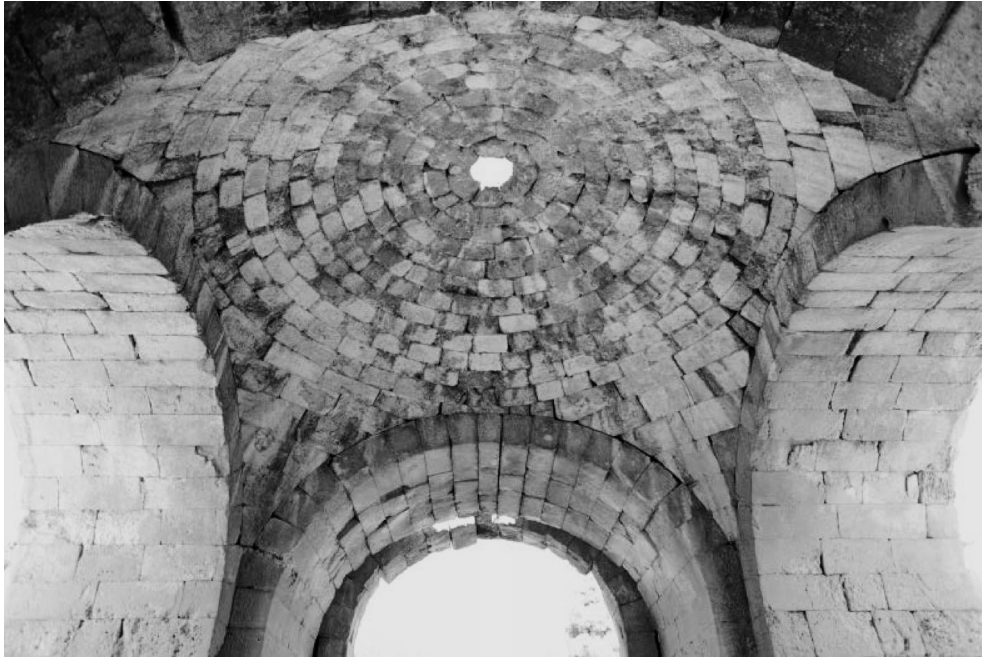
Fig. 20 Jerash, domical vault with pendentives of West Baths, looking from the south to the north
