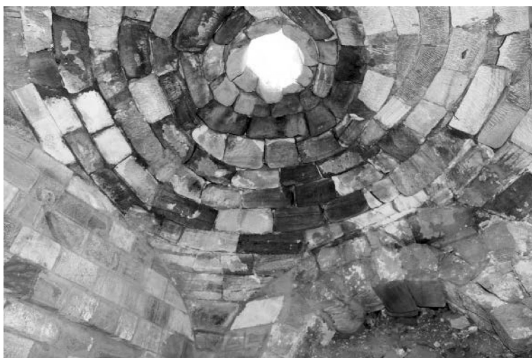
Fig. 5 Petra, domical vault with pendentive of the circular chamber of the Baths
