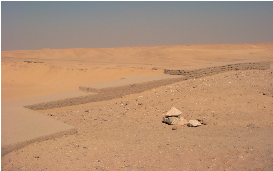
Fig. 11 After completion of the conservation (semi-reconstruction) work
