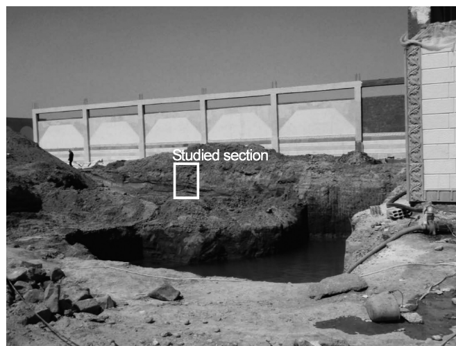
Fig. 4.4 Studied section in the factory under construction (Site 2).
