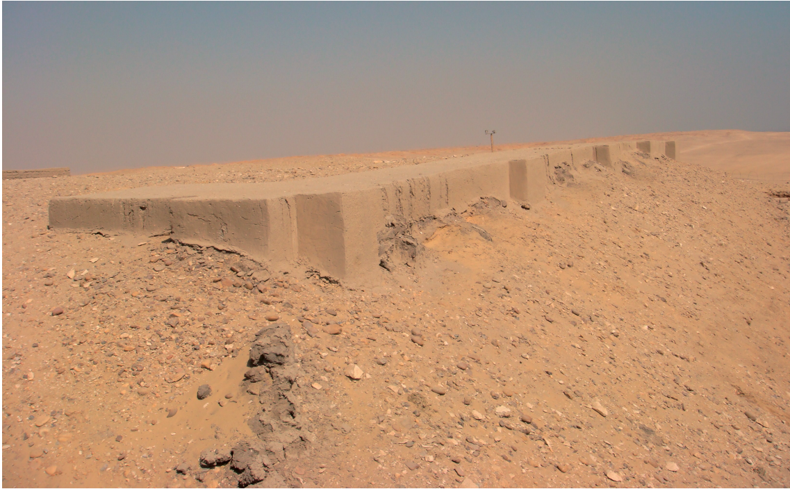
Fig. 12 After completion of the conservation (semi-reconstruction) work
