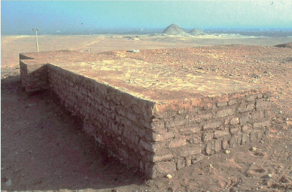
Fig. 10 Inside of the wall was filled with sand and then covered with mud
