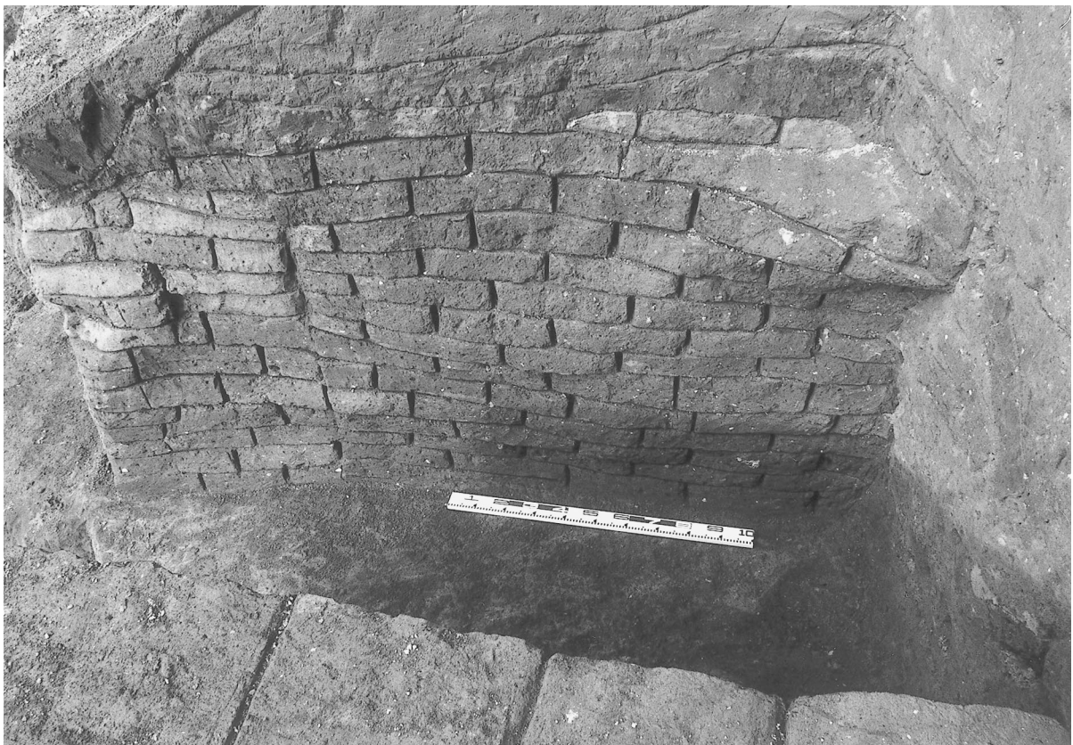
b. Entrance-like structure of Level 2 in Trench 5, from the west
