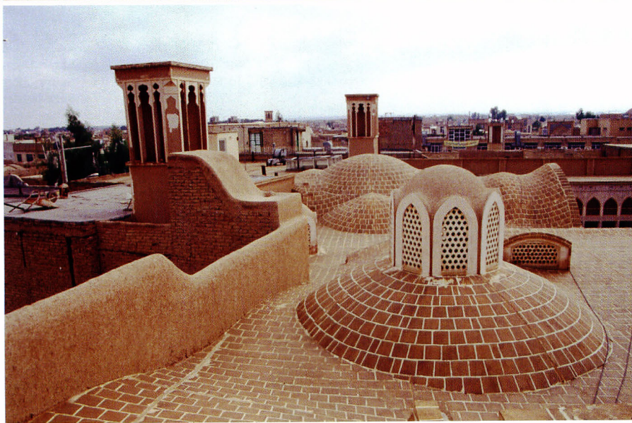
b: The climatic adaptation of the earthen architecture in Iran has produced the famous tradition of the wind towers or "badguirs" which can be still observed in the desertic region of Yazd (Central Iran) and in numerous other regions suffering of a very hot climate in summer. Here, such bioclimatic devices are observed on the roofs of the "Brugerdaha house", located in Kashan, one of the jewels of the Kajar architecture (end of the XIX th Century and beginning of the XX th Century).
