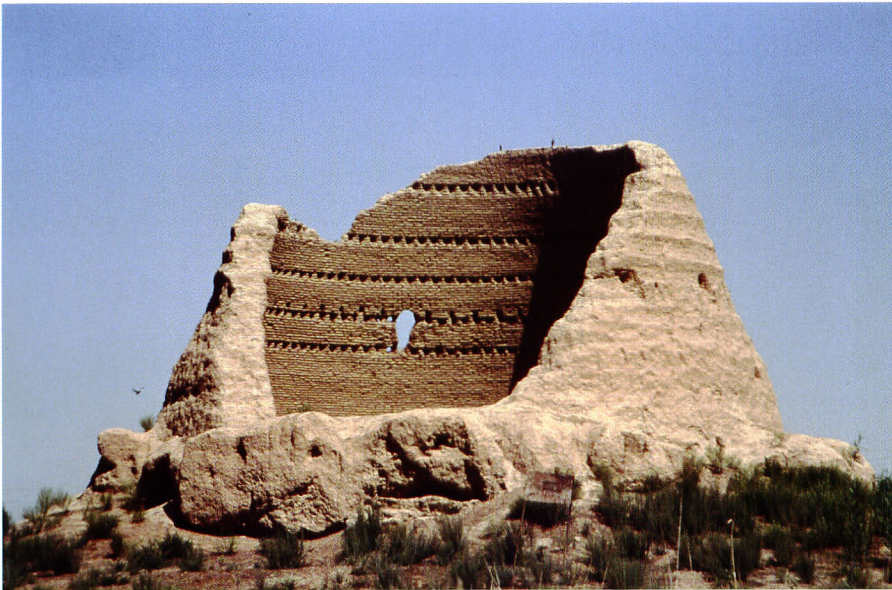
a: On the same site of Ancient Merv, visitors can observe an impressive structure built in unbaked earthen bricks, a ice house. This tradition of such big structures used for storing the snow, the ice and the cold water in big tanks deeply embedded in the ground is one of the permanent feature of the vernacular architecture of the Central Asian region.
