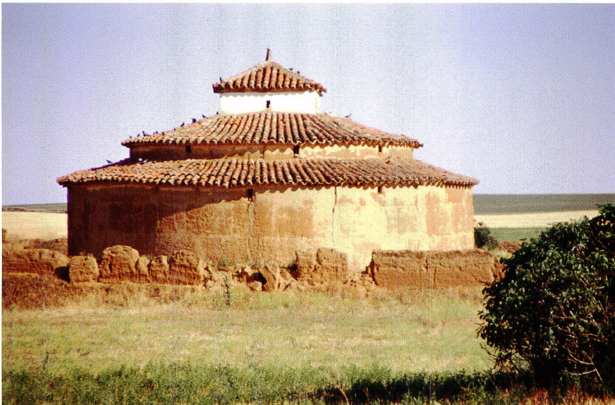
b: The presence of numerous pigeon towers, or “palomares” is one of the typical feature of the traditional rural landscape of the region of “Tierra de Campos”, Northern Spain. This tradition of round-shaped pigeon towers in “ pisé ” (“ tapial ”) is one of the most achieved in Europe where some other nice examples can be still observed in France, in the Saone River Valley (North of Lyon) or in the region of Aquitaine (South-West of France), where these “ pigeonniers ” are built in adobe.
