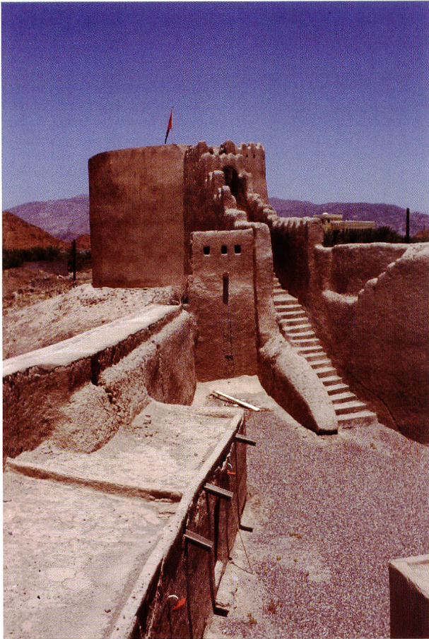
a: The Sultanate of Oman testifies of a very nice earthen architecture built in unbaked earthen bricks which have been traditionally conical-shaped and recently evolving to the common rectangular shape. This traditional earthen architecture of the Sultanate covers numerous examples of Forts with massive outer defensive walls and towers, or “ borjs ”, and a nice tradition of outdoor and indoor plastering in “ sarooj ” (natural lime) or “ juss ” (gypsum) as well as earth and straw. Here the Fort of Bid Bid, on the road from Muscat to Nizwa. The Fort of Bid Bid has been restored during the 80’s of the last XX th Century by the Ministry of National Heritage of Culture which has recently conducted new restoration works valorising the aesthetic of the traditional renderings.
