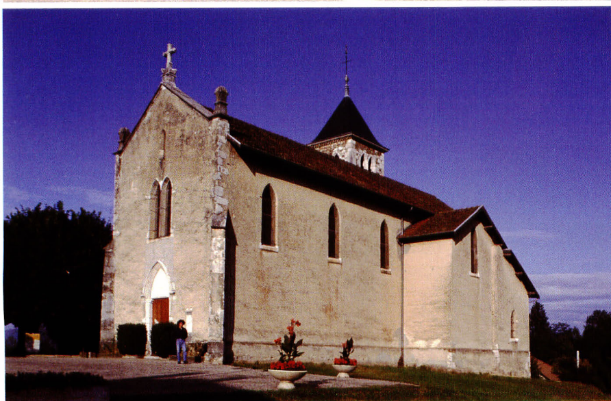
c: A rare and nice example of a Christian church built in “ pisé ”, plastered with a thin lime distemper, in Isere, village of Charancieu located around 30 km north Grenoble. This church has been built at the middle of the XIX th Century. All walls, excepted those of the bell tower are in “ pisé ”.
