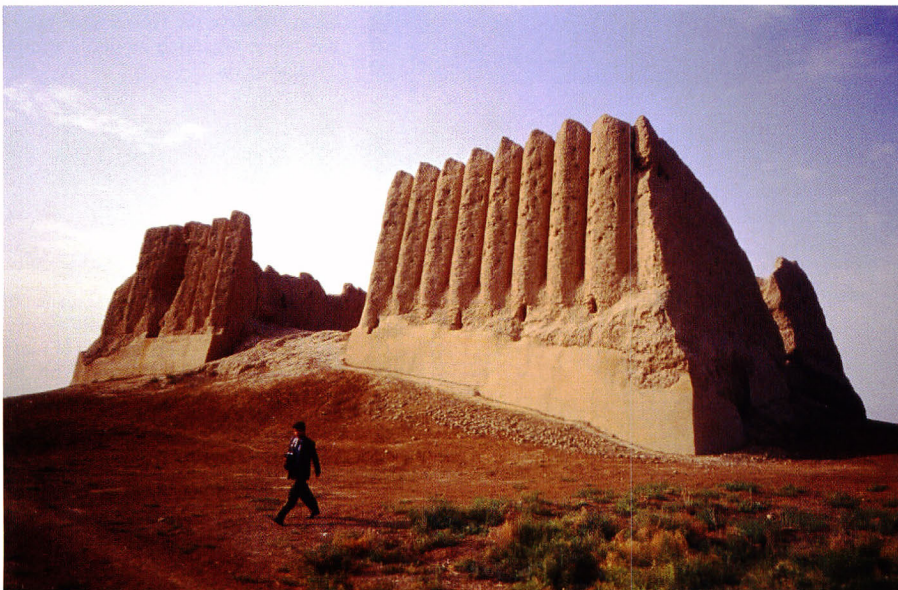
b: In Turkmenistan, the famous medieval site of Ancient Merv which has been entered on the List of the World Heritage of UNESCO in 1998. The original architectural design of the outer walls of the “ Great Kyz Kalā ”, built in unbaked bricks during the XI th and the XII th Centuries A.D. is today known as a “ corrugated ” structure the shape of which having been compared with other structures of a similar type existing in Iraq.
