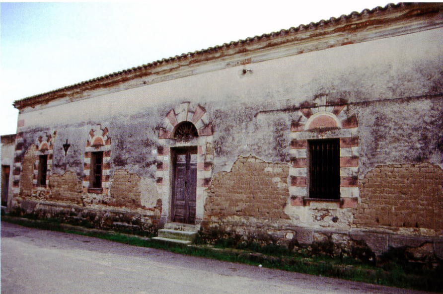
b: Typical house in unbaked earthen bricks, “ladriri” or “mattoni”, in southern Sardinia, region of the “Campidani”, village of Riola Sardo. In this region, numerous villages are built in earth and a programme for their conservation, restoration, rehabilitation and maintenance, associated to a revival of the earthen building technology has been recently launched under the guidance of the University of Cagliari in close collaboration with the municipalities. This tradition of the unbaked earthen brick traces back to Greek, then Punic (site of Tharros) and Roman times.
