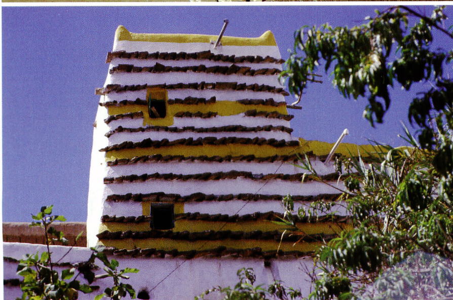
c: An other typical and nice tradition of earthen architecture in Saudi Arabia, here built in unbaked bricks. In this region the climate is not only dry but also humid with some hard and very devastating rains and flooding. To protect their houses, traditional builders have included in the façades of the houses layers of salient stones which are pushing out the rain water. On the other side, during the hot season, these stones are also maintaining a projected shadow which contributes to the cooling of the walls and the bioclimatic conditioning of the houses.
