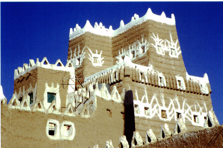
b: Typical earthen people’s housing in the South of Saudi Arabia, region of Najran. These constructions are made of successive “ cob ” layers (stacked packs of plastic earth). The desert climate of this region authorizes a basic protection of the more exposed parts of the structures, the top of the walls and the outer reveals of the bays that are generally plastered with natural white lime which are regularly maintained.
