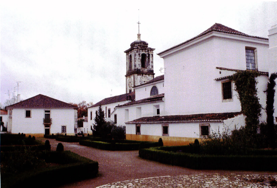
b: The construction in “ pisé ” (“ taipa ”) is a permanent feature of the history of architecture in Portugal. Here the palace of the ducal City of Villa Viçosa.
