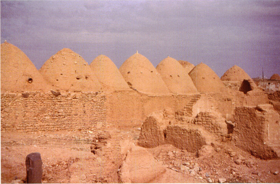
a: A traditional village in the region of Aleppo, Syria. Here, the earthen building culture testifies of a traditional roofing system in corbelled conical cupolas. Such structures are now very rare but this know how is tracing back to very old times as it has been confirmed by some graffitis which have been found in Niniveh (Assyrian times) evocating the rural people's of this period.
