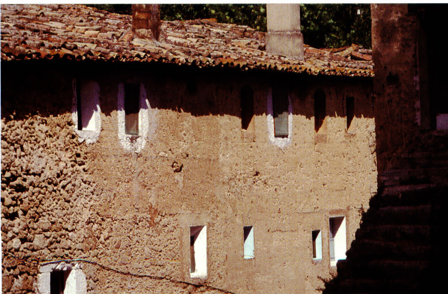
c: Eastern Mediterranean seaside of Spain, inland region of Catalonia, around Barcelona. Numerous villages are built in rammed earth or “tapial” which is no more a living building culture.
