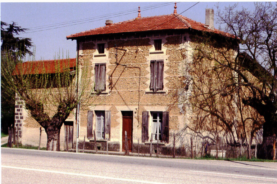
b: A typical village house in “ pisé ”, built at the beginning of the XX th Century, with reveals in concrete, located in the northern part of Dauphiné, region of Isere, South-East of France. Most of these houses are not plastered though the local climate is very rainy in Spring and Autumn. The main front façades of wealthier houses are sometimes decorated with layers of burnt bricks and river pebbles.
