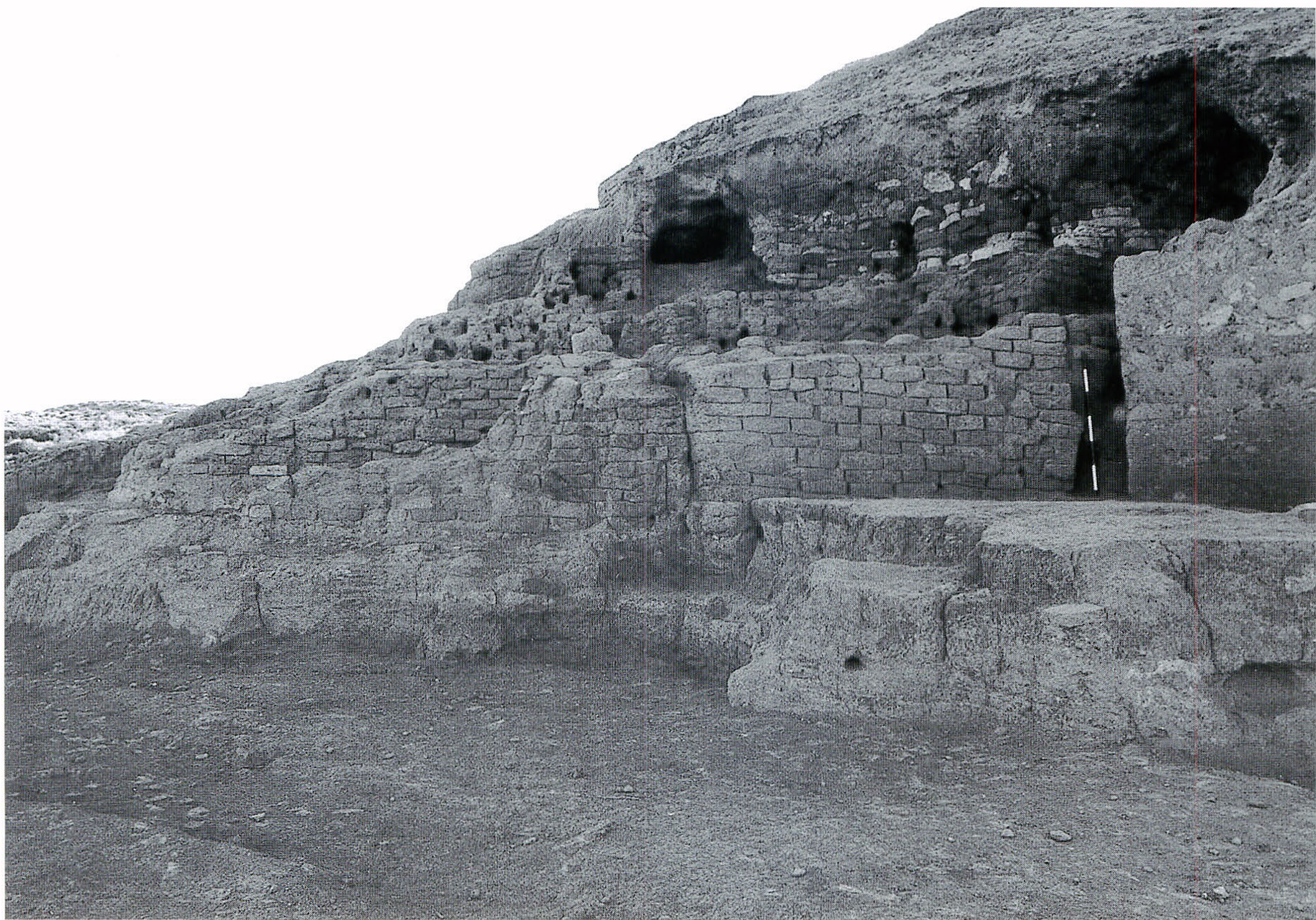
a. Huge Wall 1 seen from the west
