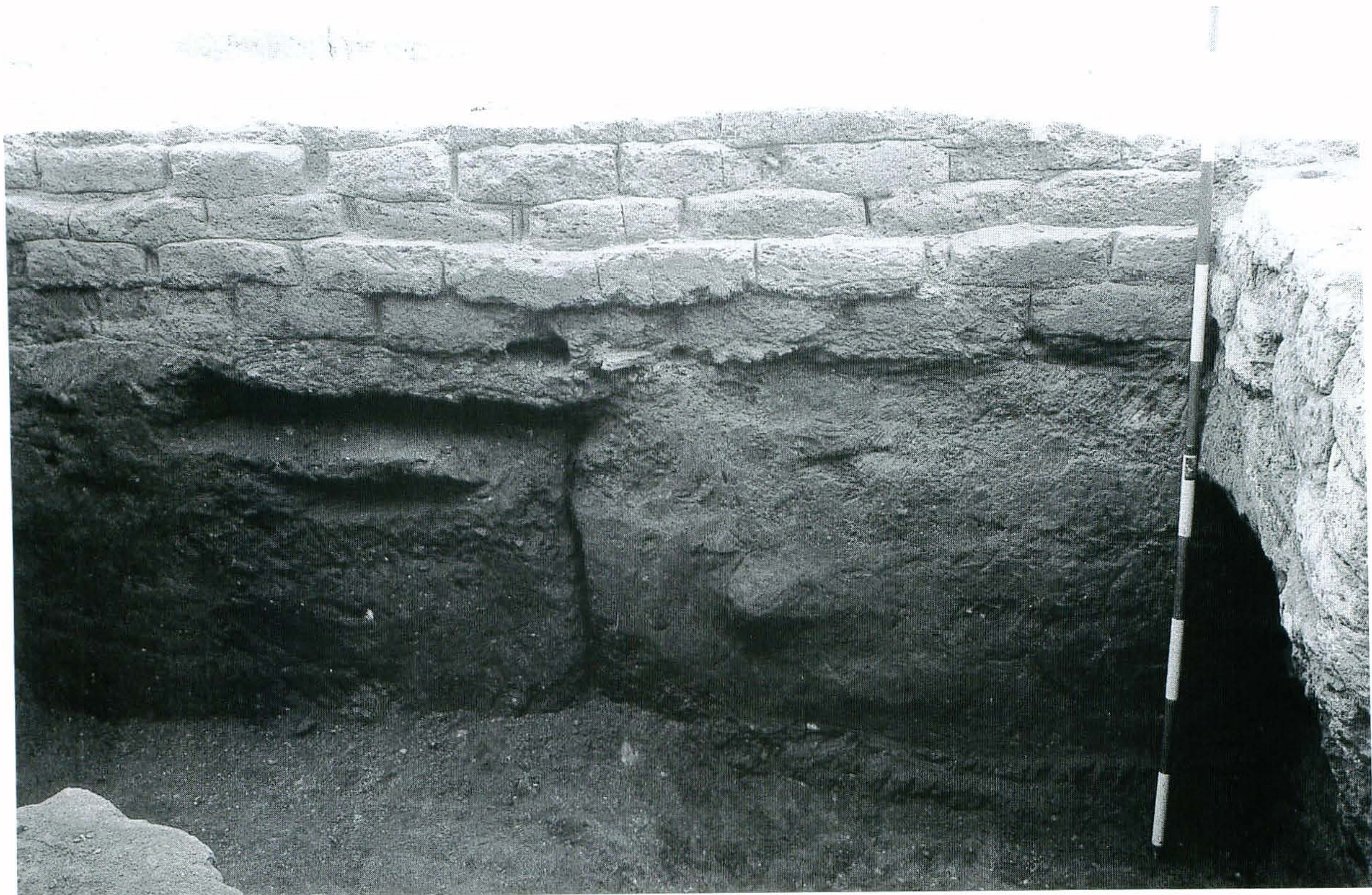
a. Inner surface of Wall 3 (Level 9) and Wall 4 (Level 10), with coating on Wall 4 not uncovered
