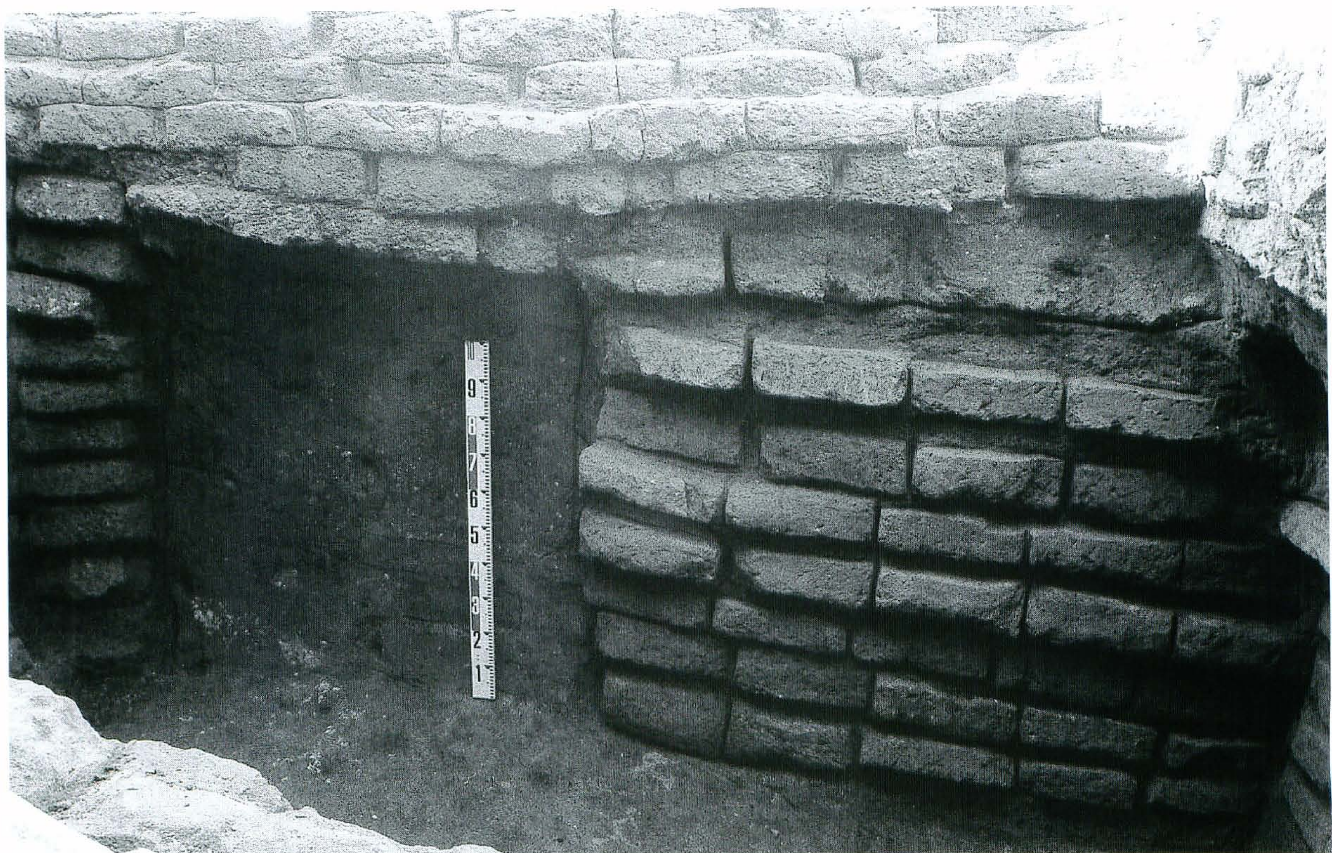
b. Inner surface of Wall 4 (Level 10) with coating uncovered
