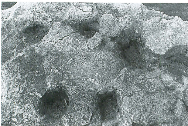
a) Holes in the firebars (from the south)
