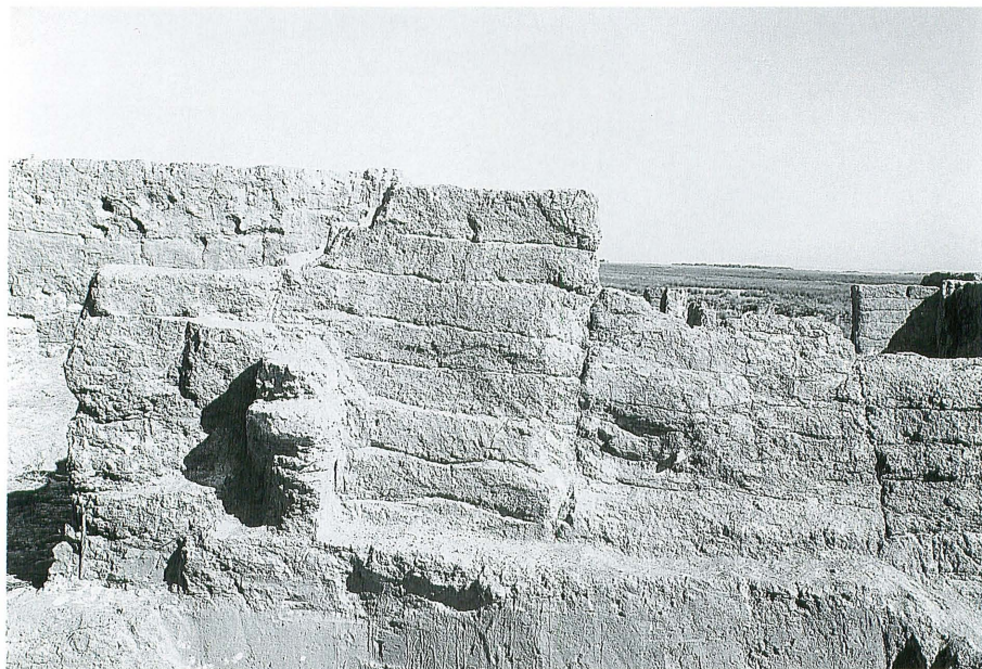
a) Closed entrance to Room 13b (from the southwest)
