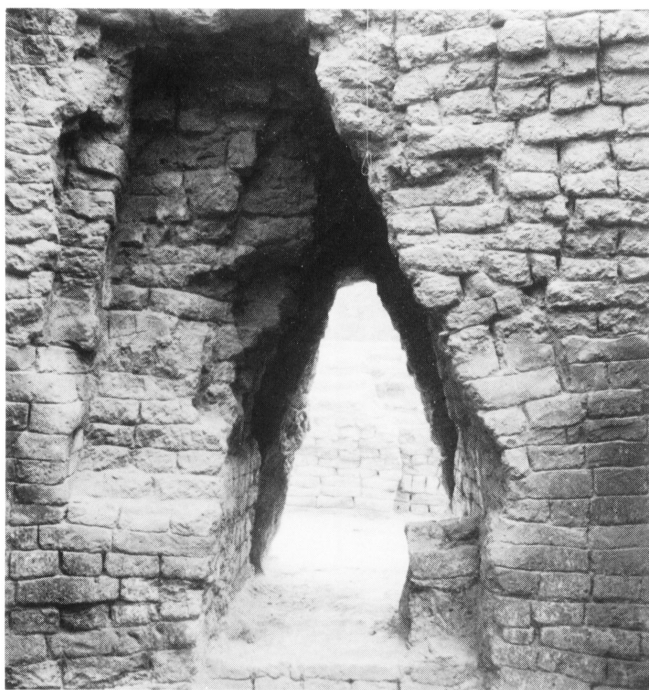
1 VII層 迫出穹窿構造 Corbeling Vault Structure, Level VII
